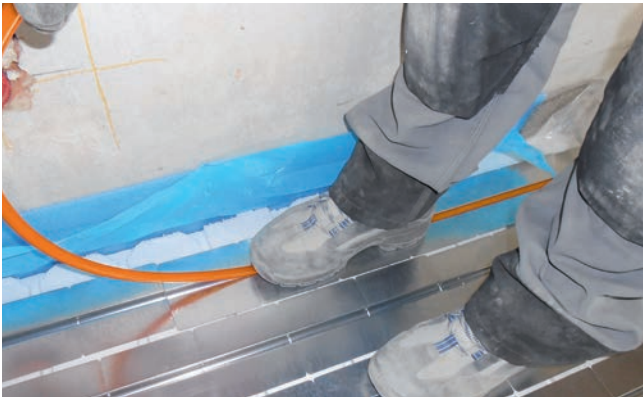
Laying of heating pipes
