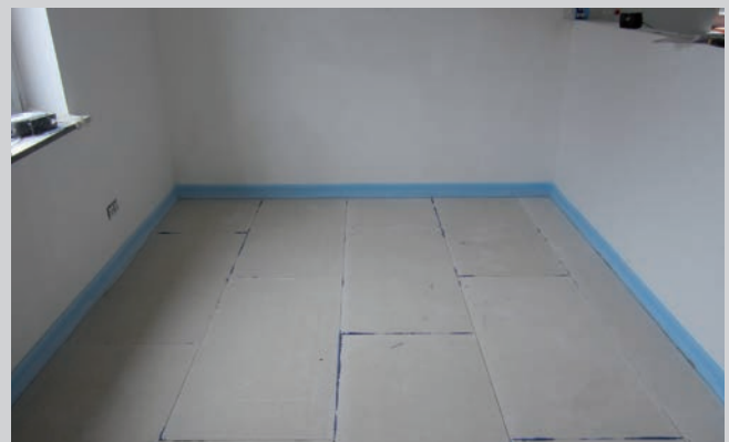
Finished dry elements
