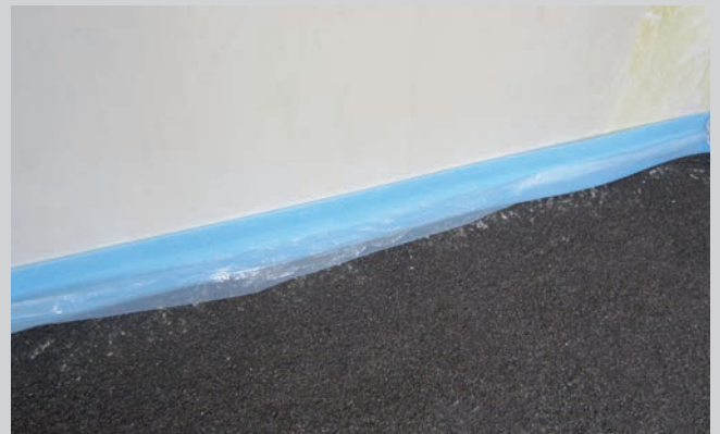
Laying of edge insulation
