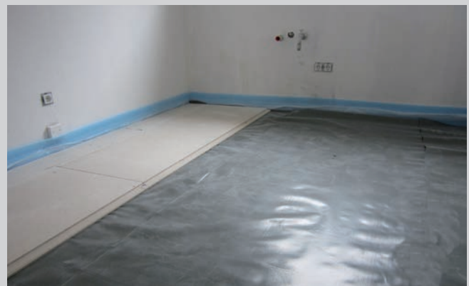
Depending on manufacturer's specifications for prefabricated screed the mounting of a release film may be necessary.
