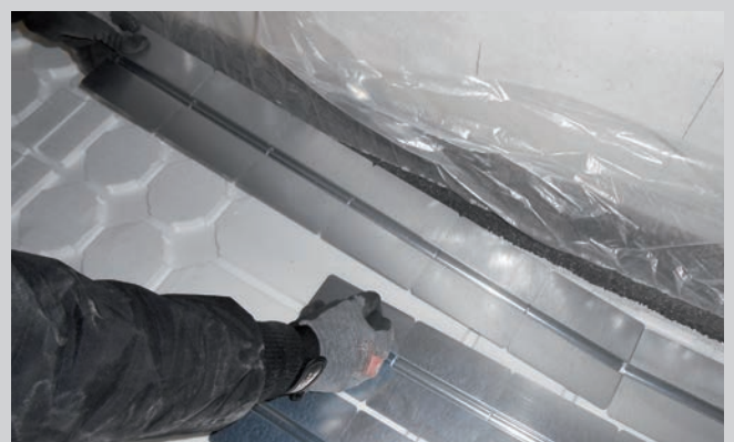
Installation of heat conducting steel sheets
