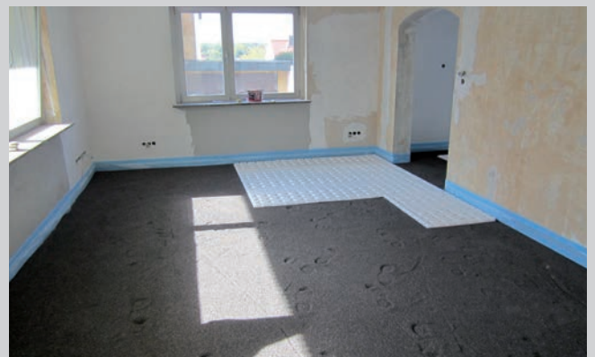
Laying of system element
