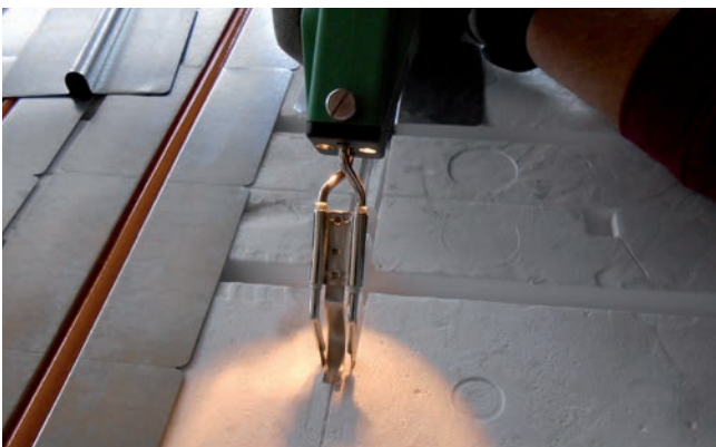
Required extra pipe channels such as connecting pipes are made by filament cutter.
